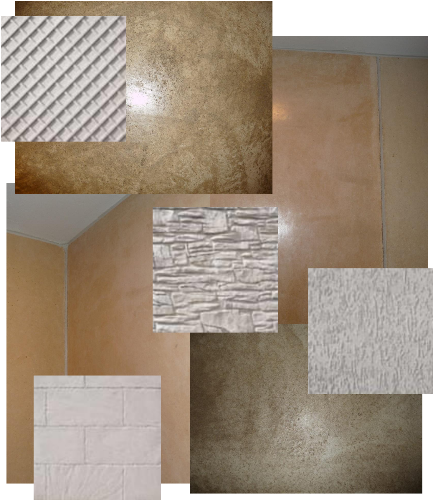
FIG. 6 – SIMPLE EXAMPLES of PRECAST AS-CAST FINISHES – PIGMENT AND FORM LINER
